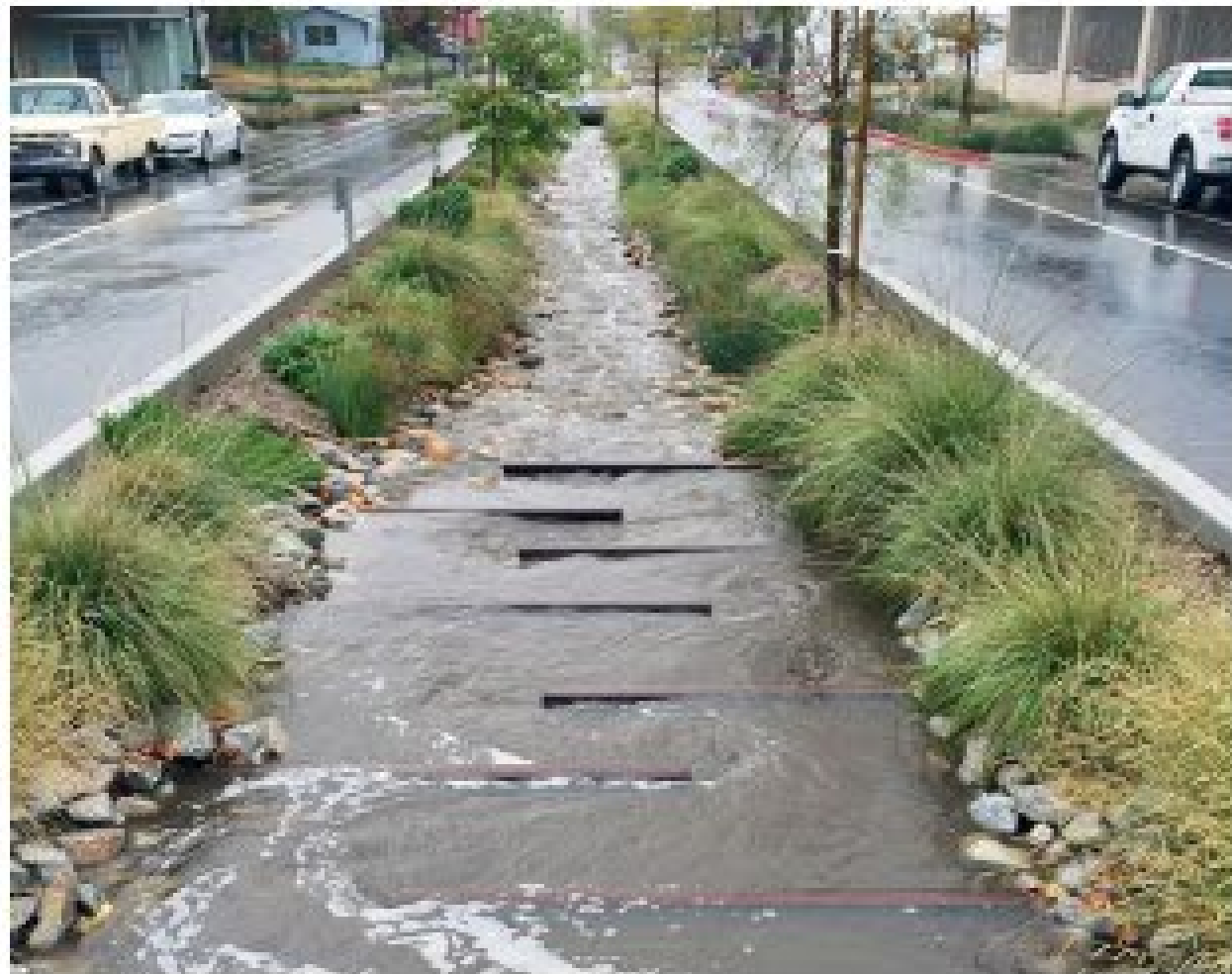
21st Street Redesign, Paso Robles, California Photo credit: MIG/SVR
